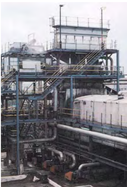
View of cane diffuser inlet
